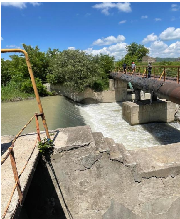
Headworks at Mashavera River
