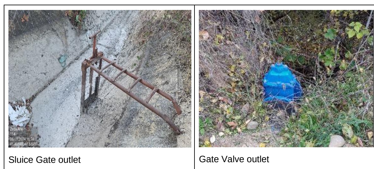
Photo 1: Existing type of Canal Outlets
