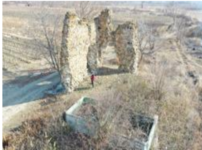
Figure 33: Nameless Tower Poor Condition
