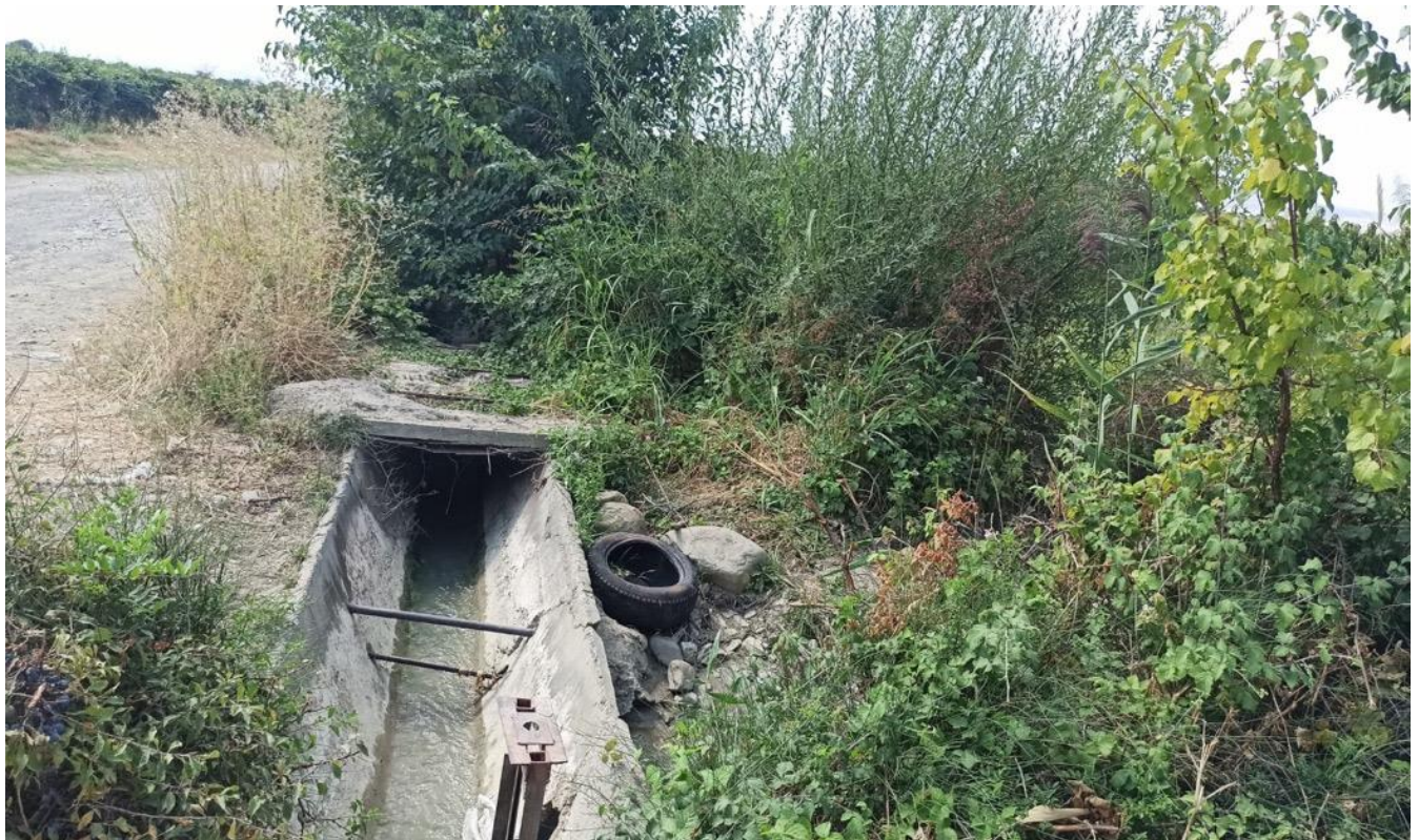
Figure 19. Available space for buried pipes and available access road; existing channel that will be replaced with buried pipes
