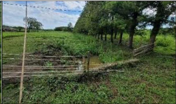
(f) Secondary Drain (S-K-2-3-2)
