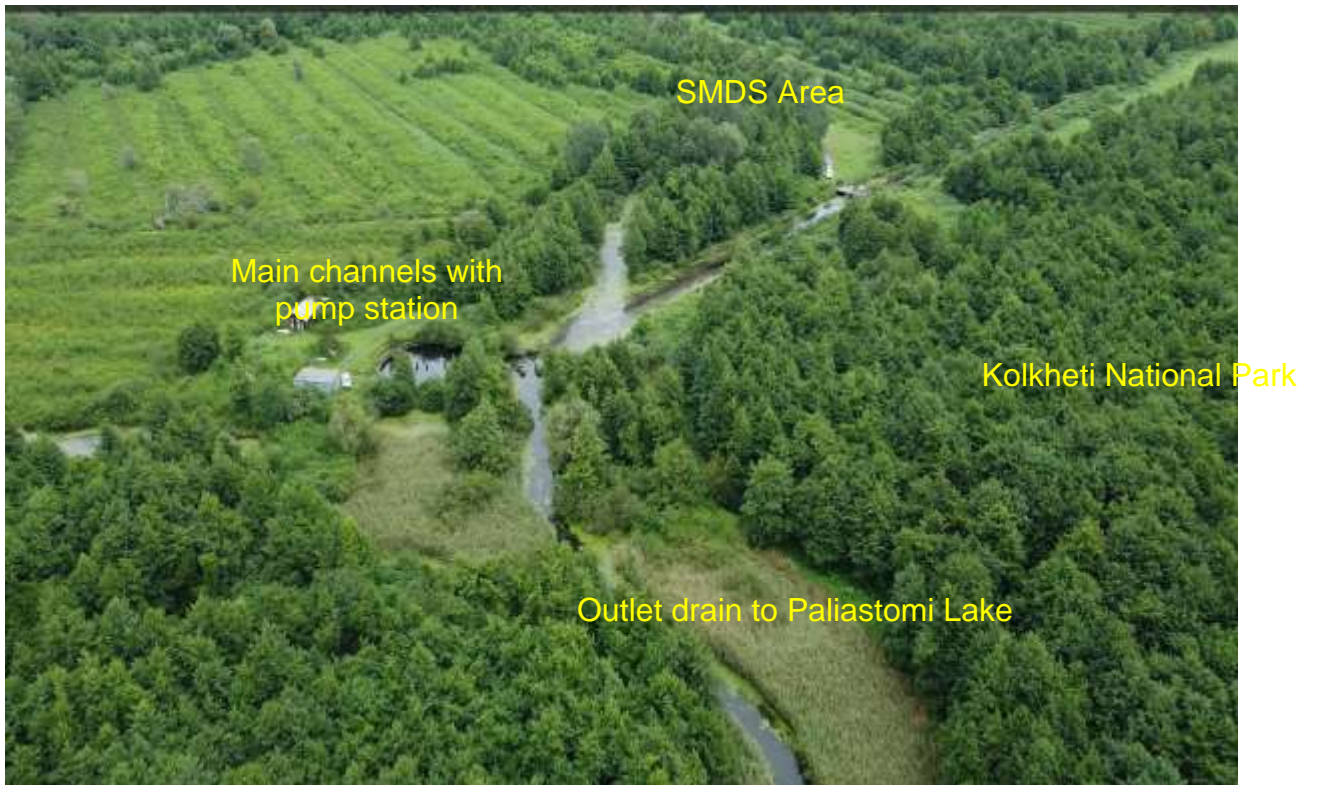
Figure 10: A view of the drainage water flowing to wards Paliastomi Lake
