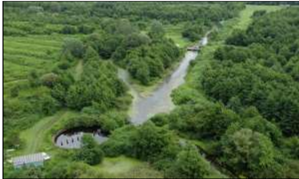
(e) Main Drain (S-K-2)
