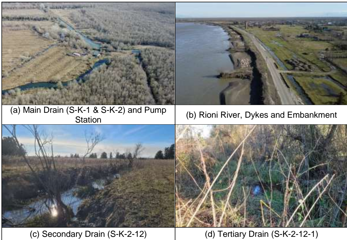
Photo 3: Third Field Visit (22 January 2025)
