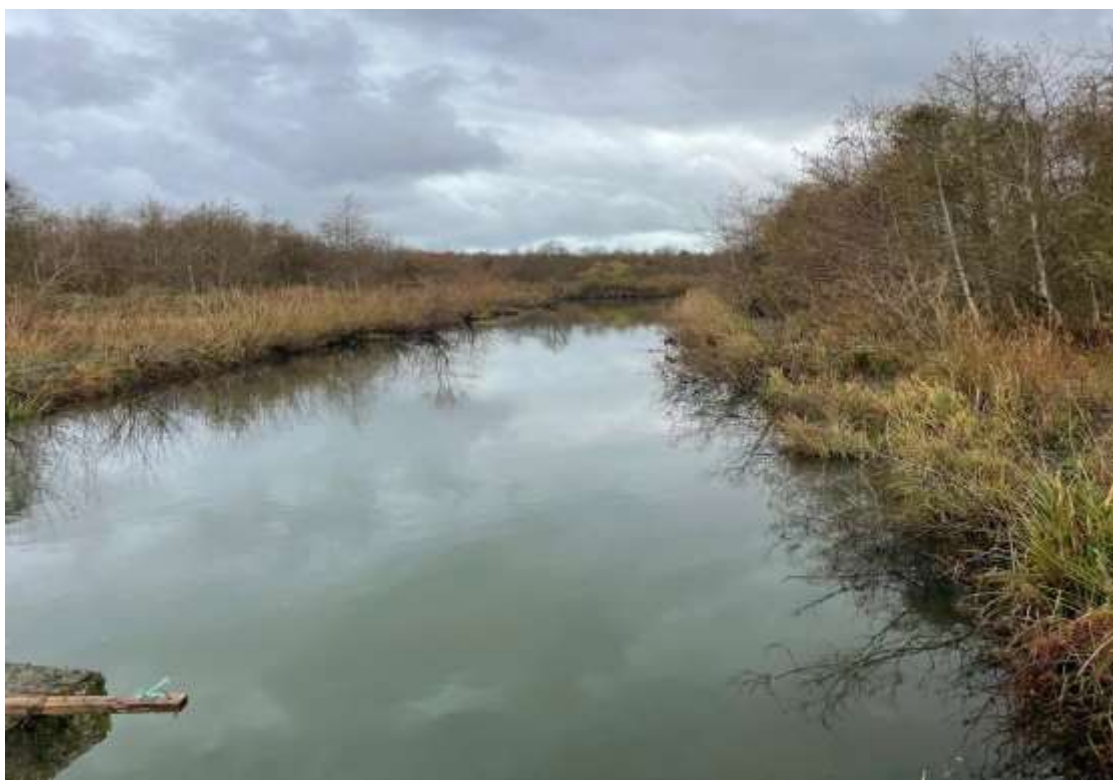
Figure 2: Main Channel condition of the existing drainage scheme
