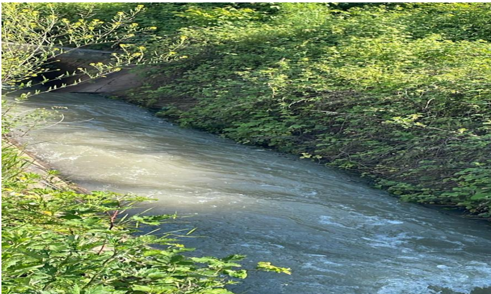
Cyphone on the main Canal
