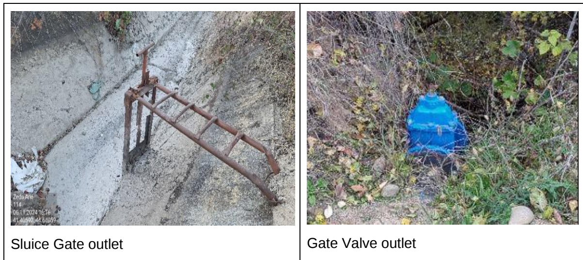
Photo 1: Existing type of Canal Outlets
