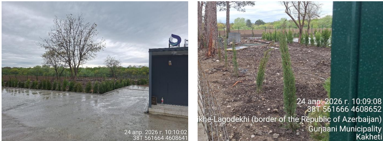
Figure 21. Planting and landscaping works at the new GA building
