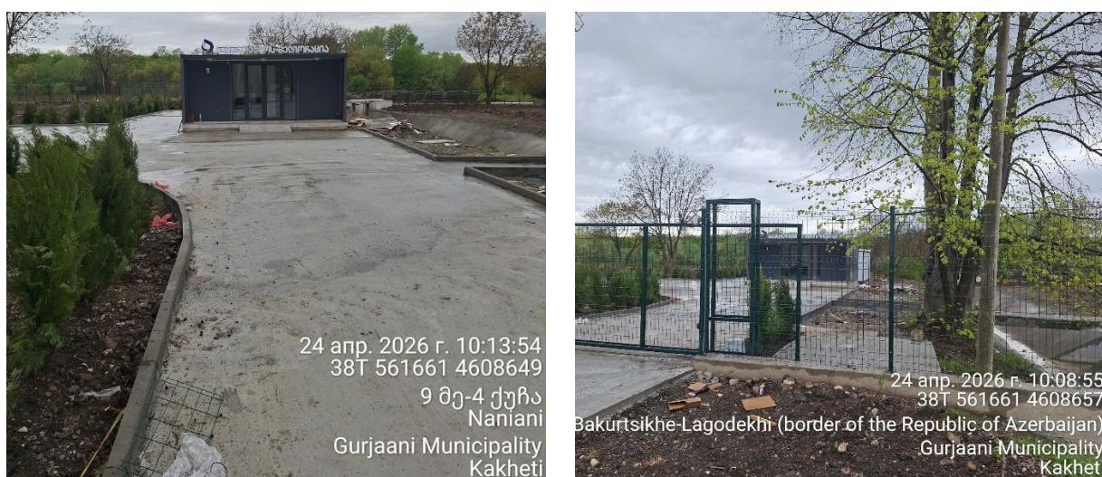
Figure 9. GA New Service Center Building (April, 2026)
