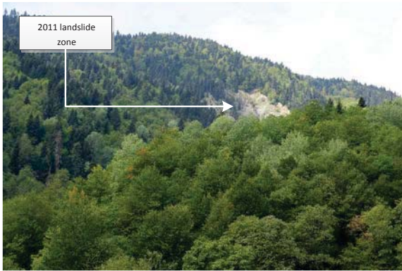
Lekverari gorge - zone exposed to landslide risk
