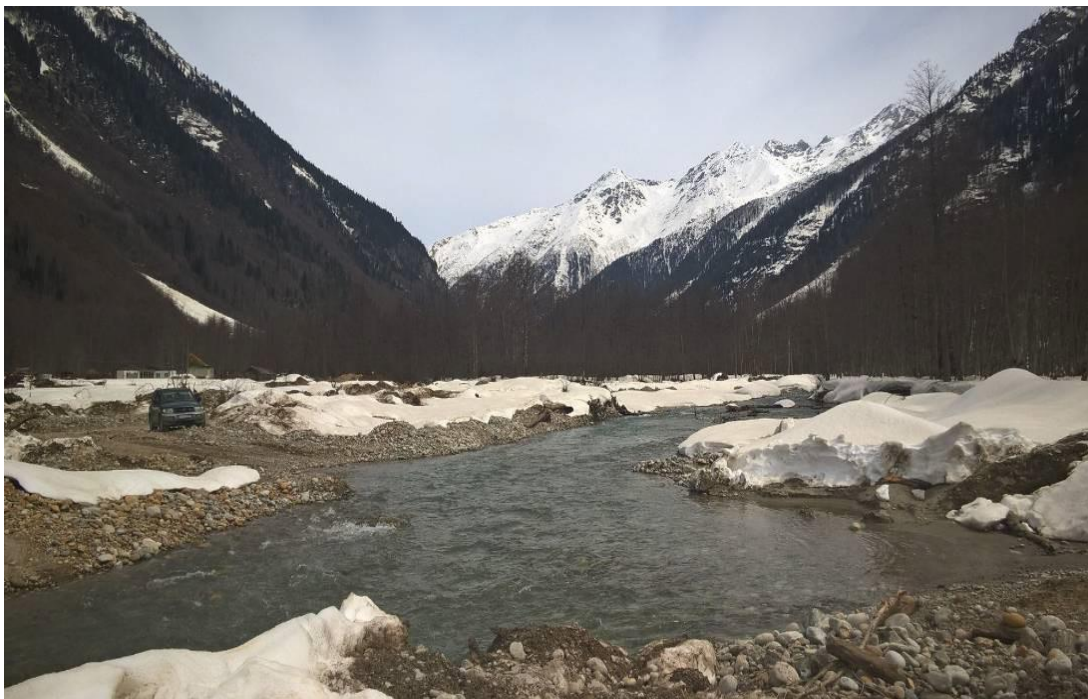
Photo 1.1: a view of Dam area.
