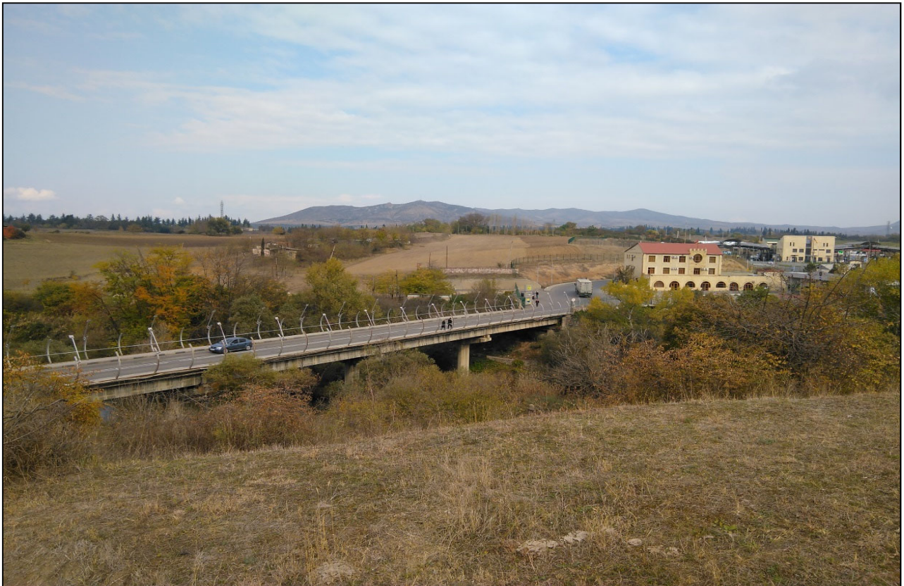
BAGRATASHEN BRIDGE - NORTH VIEW
