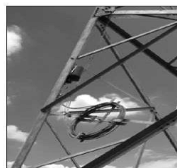
Installation on tower
