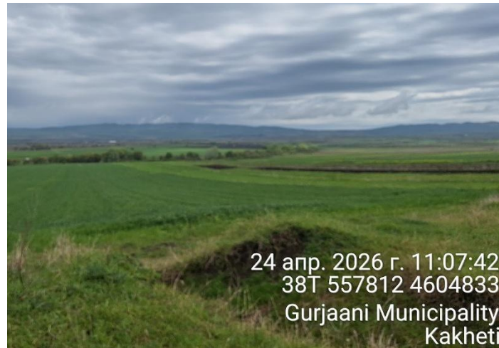
Figure 12. Unauthorized artificial trench dug by locals, causing damage to the degraded G-42 canal and the adjacent local unpaved road (April, 2026)
