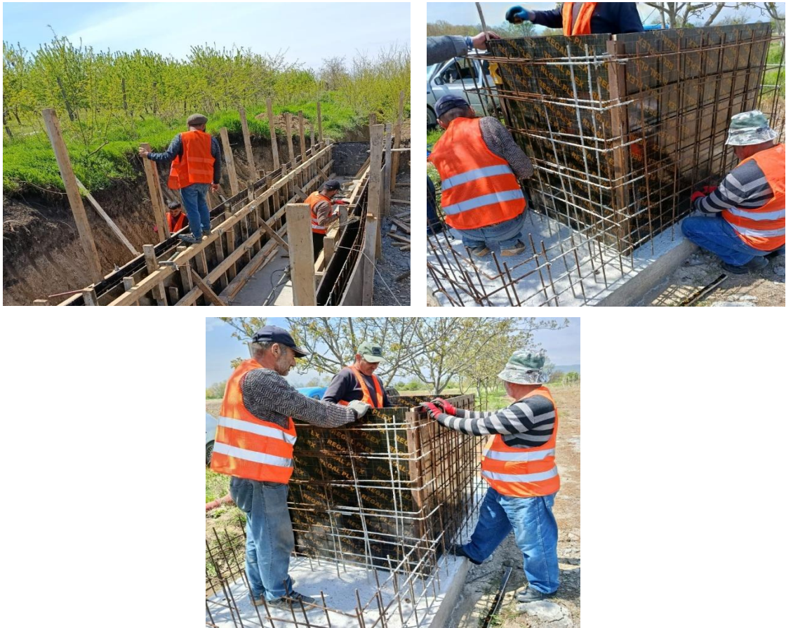
Figure 22. Work process and PPE usage practices
